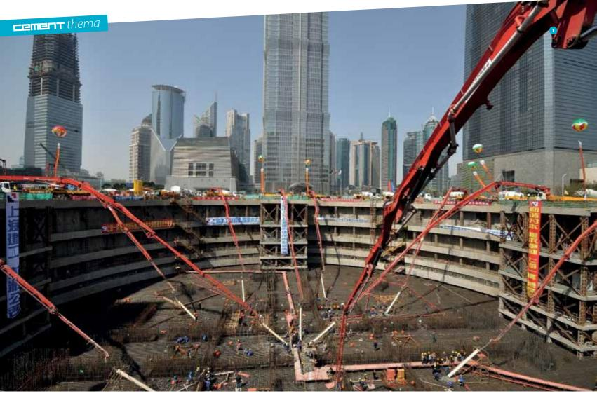
Monolithic pouring of the foundation slab of the 632 m high tower
